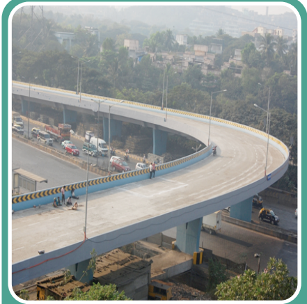
Suman Nagar Flyover-MSRDC
